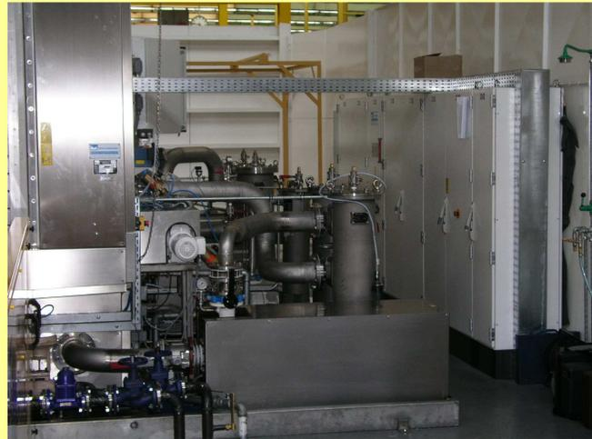
Pic. 4: Attachment: Double fine filter, enclosed pumps, control cabinet, drive motor for trolley insertion...
