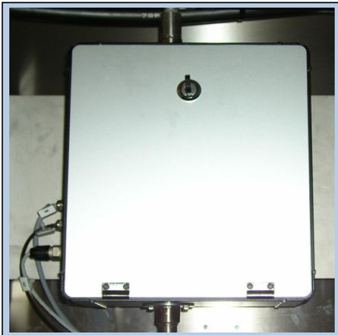
Pic. 3: Measuring cell for analysis of medium
