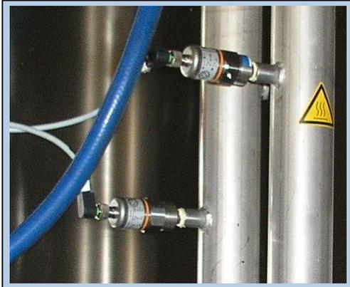
Pic. 1: Pressure sensors for pressure monitoring
